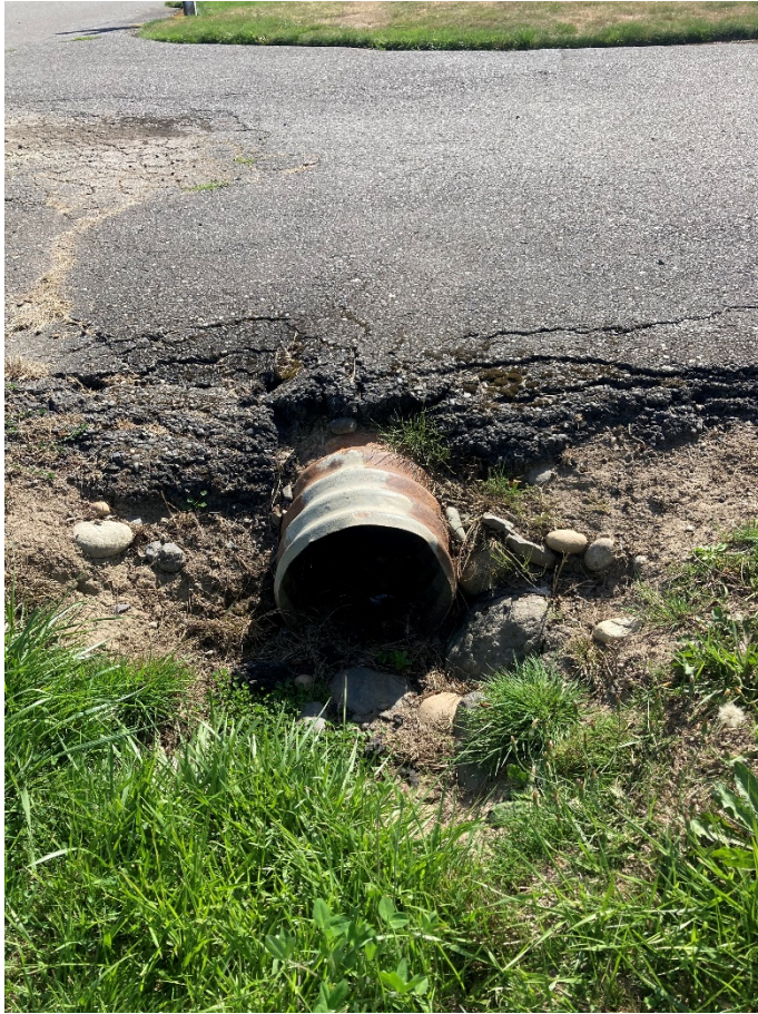
Figures 5 & 6. Road culvert (CV# 3586) under East Shoreview, east of Bay Ridge Drive. Old corrugated metal pipe, shallow cover, with a rusting bottom and some sediment and debris accumulated. Replacement is needed.
