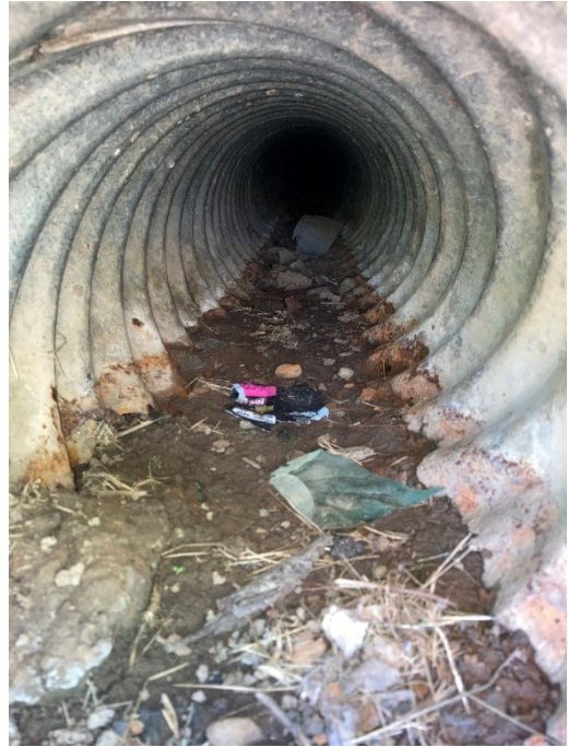
Figures 5 & 6. Road culvert (CV# 3586) under East Shoreview, east of Bay Ridge Drive. Old corrugated metal pipe, shallow cover, with a rusting bottom and some sediment and debris accumulated. Replacement is needed.
